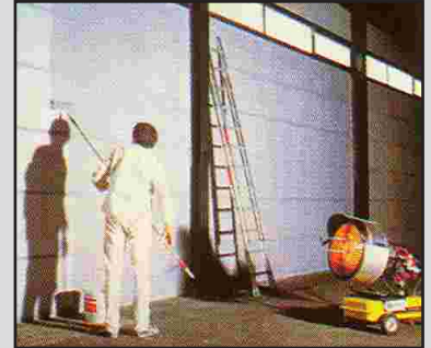
Drying and heating at construction sites.
